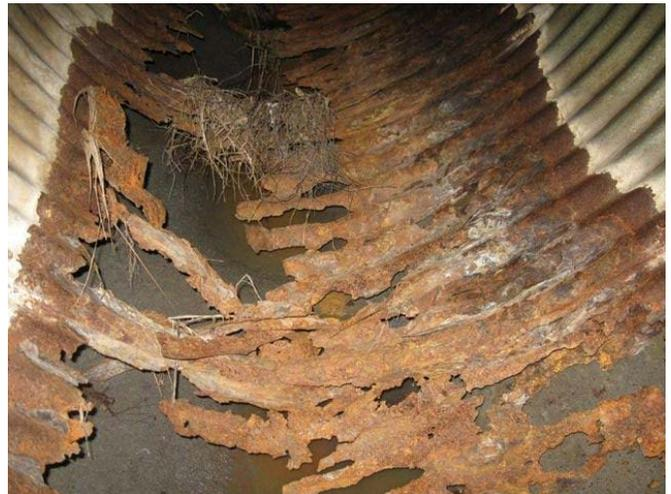
Figure 1. Severely deteriorated CMP outlet conduit. [4]
