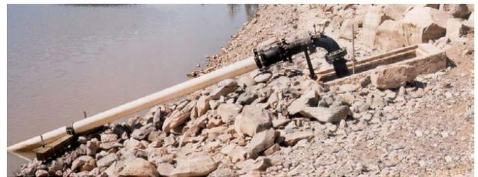
**Figure 3. Siphon used to lower the reservoir water surface through the upper entrance of an outlet works intake structure. [1]**
