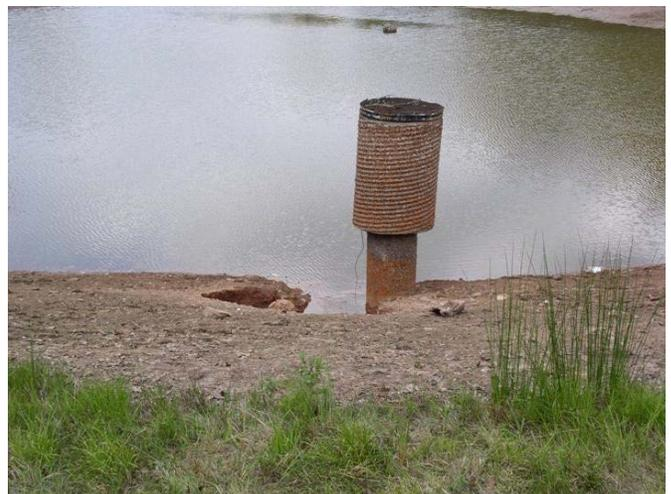
Figure 2. Typical drop-inlet structure for outlet conduit.
