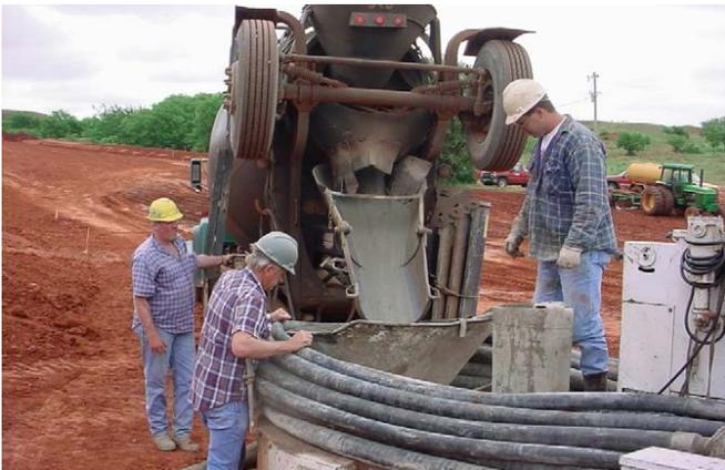
**Figure 7. Grout being delivered to the pumping truck. [1]**
