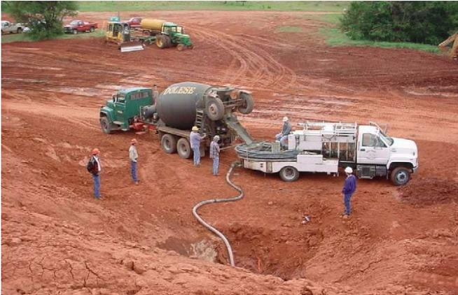
**Figure 6. Abandonment of a conduit by pumping cement grout through holes drilled from the surface of the embankment dam to depths of up to 60 feet. [1]**
