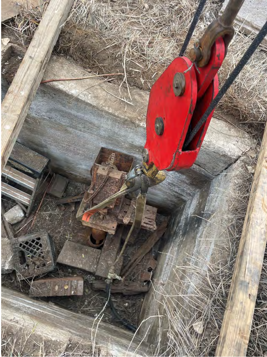
Photo 1 – Removing pump with pump rig - Pump column and shafting broke
