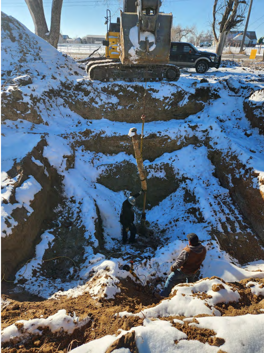
Photo 7 – Excavated and cut casing off so we could get hold of stuck column pipe
