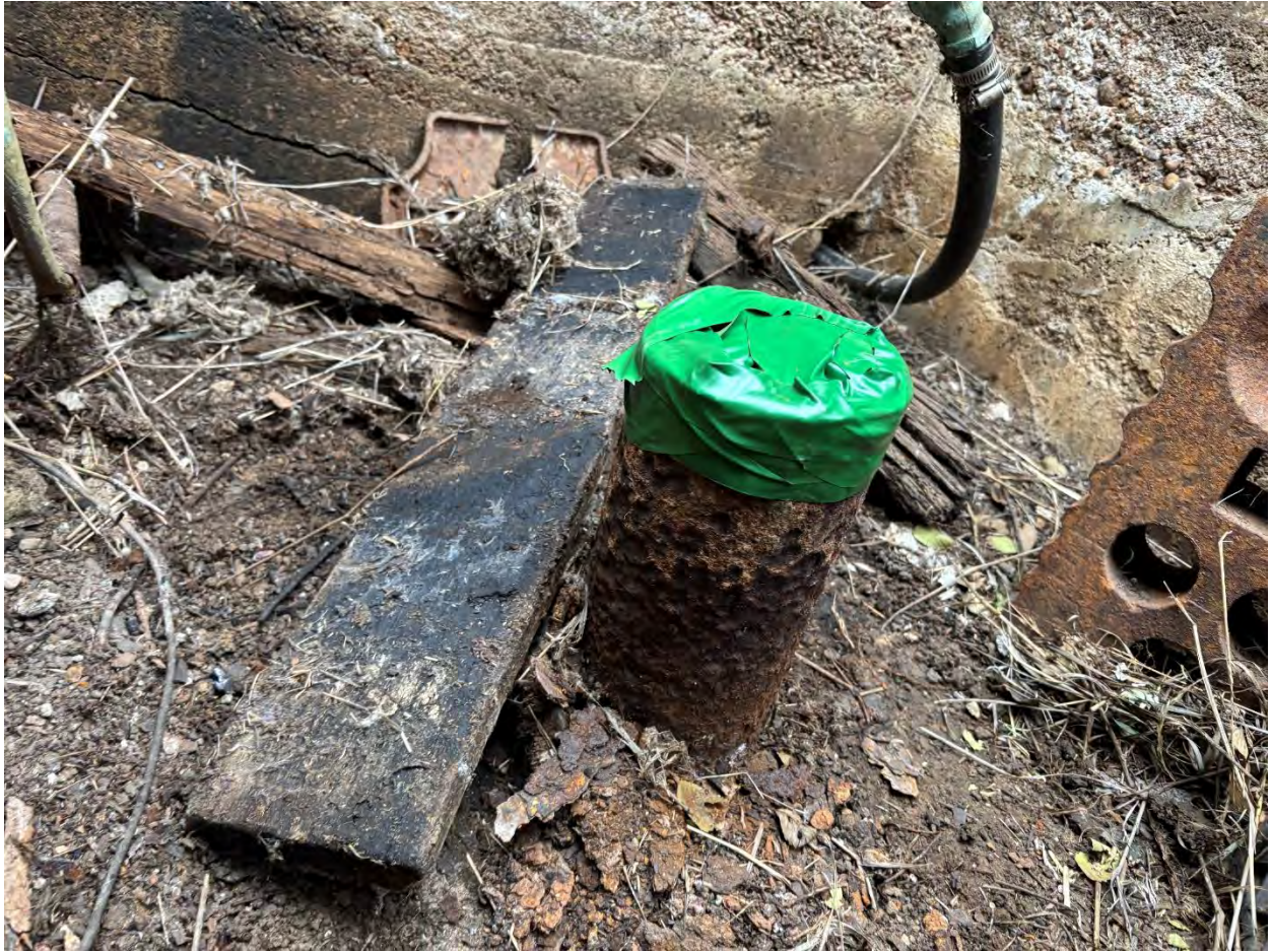
Photo 6 – Secured Casing prior to excavating to make another attempt with crane
