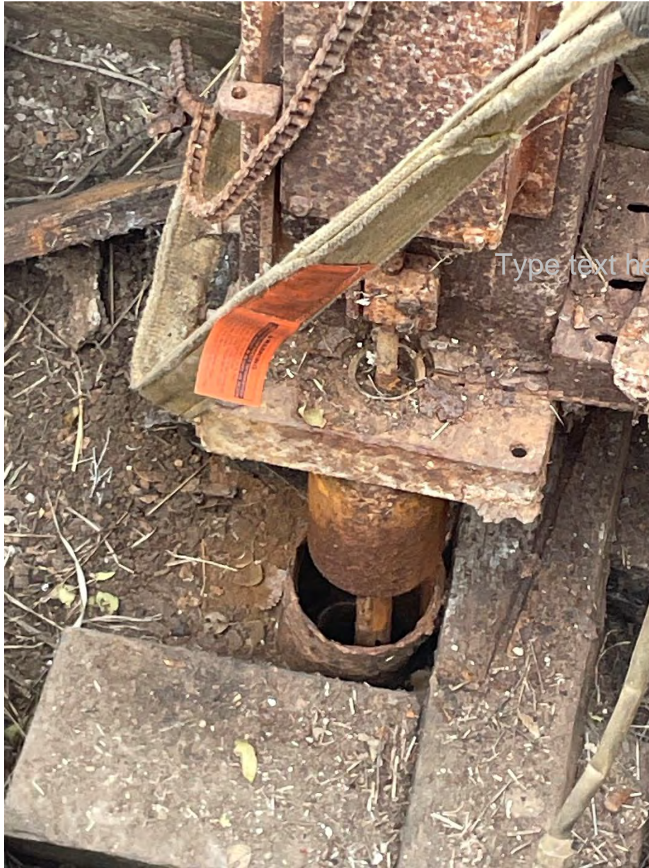
Photo 2 – Pulling Head Off – Pump Broke
