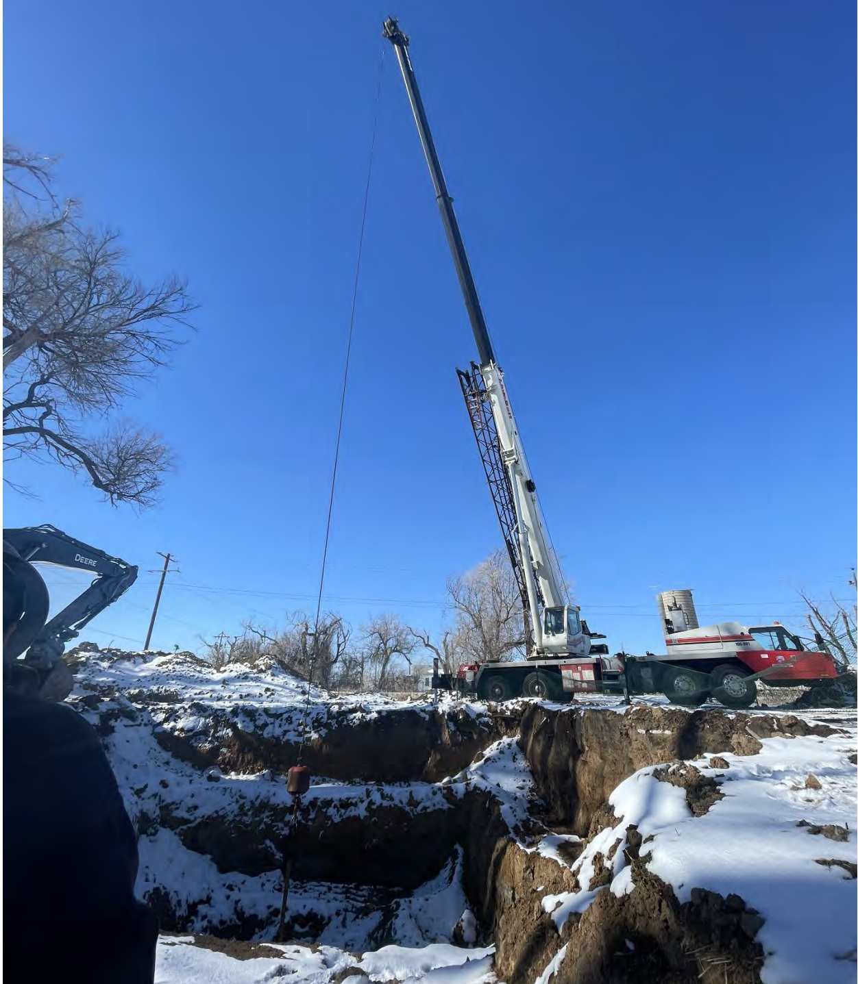
Photo 8 – Crane pull – came up approximately 36” and stuck solid – would not go up or down
