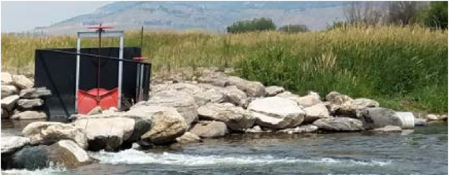
Example of a Cross-Vane/irrigation head gate-sediment sluice
