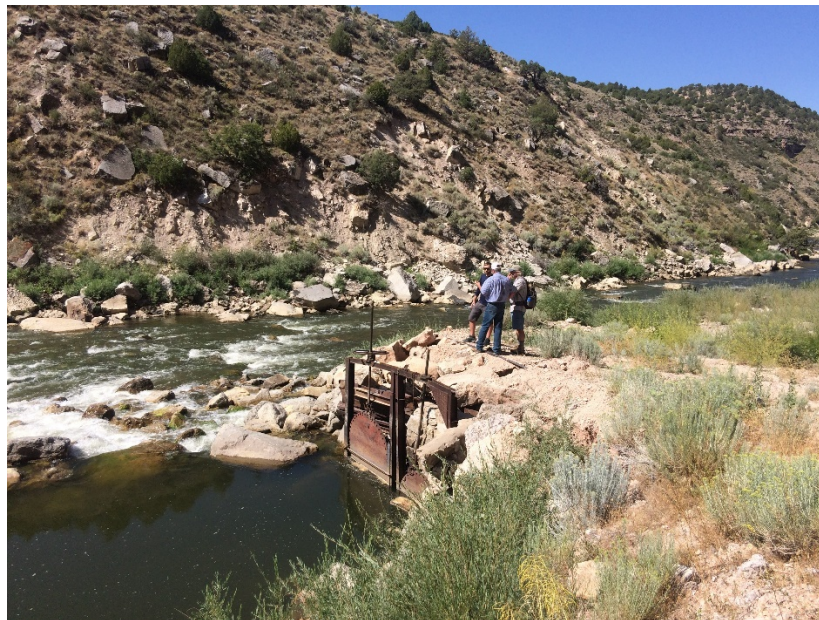
Maybell diversion and malfunctioning headgates, October 2020
