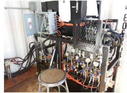
Figure 3 - After construction - new outlet controls
