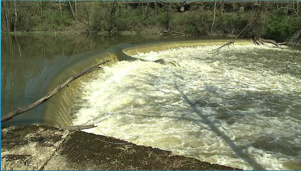
MCDONALD STEEL MILL DAM GIRARD, OHIO
