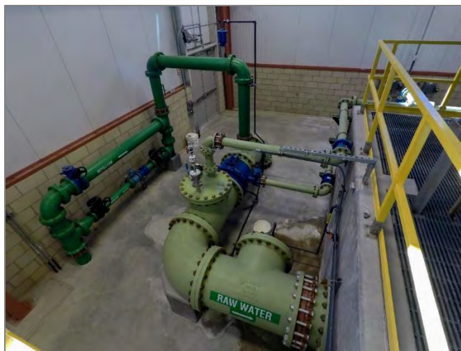
Pretreatment Chemical Injection and Jet Mixing Piping
