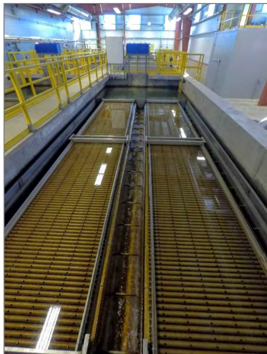
Plate Settlers in the West Sedimentation Basin
