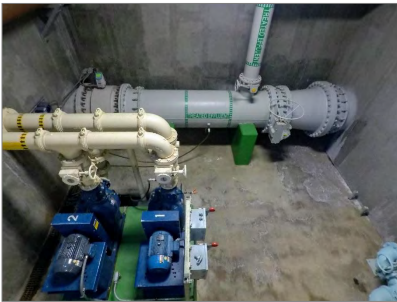
Treated Effluent Leaving the Disinfection Room
