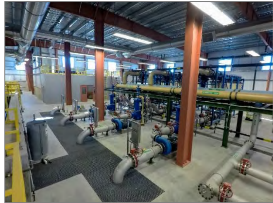
Pall Microza Membrane Filtration System
