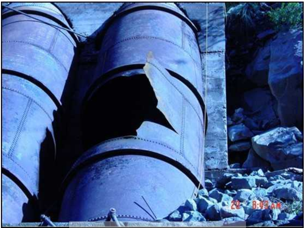
PENSTOCK RUPTURE DAMAGE
