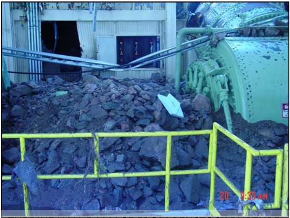
TURBINE HALL DAMAGE FROM PENSTOCK RUPTURE
