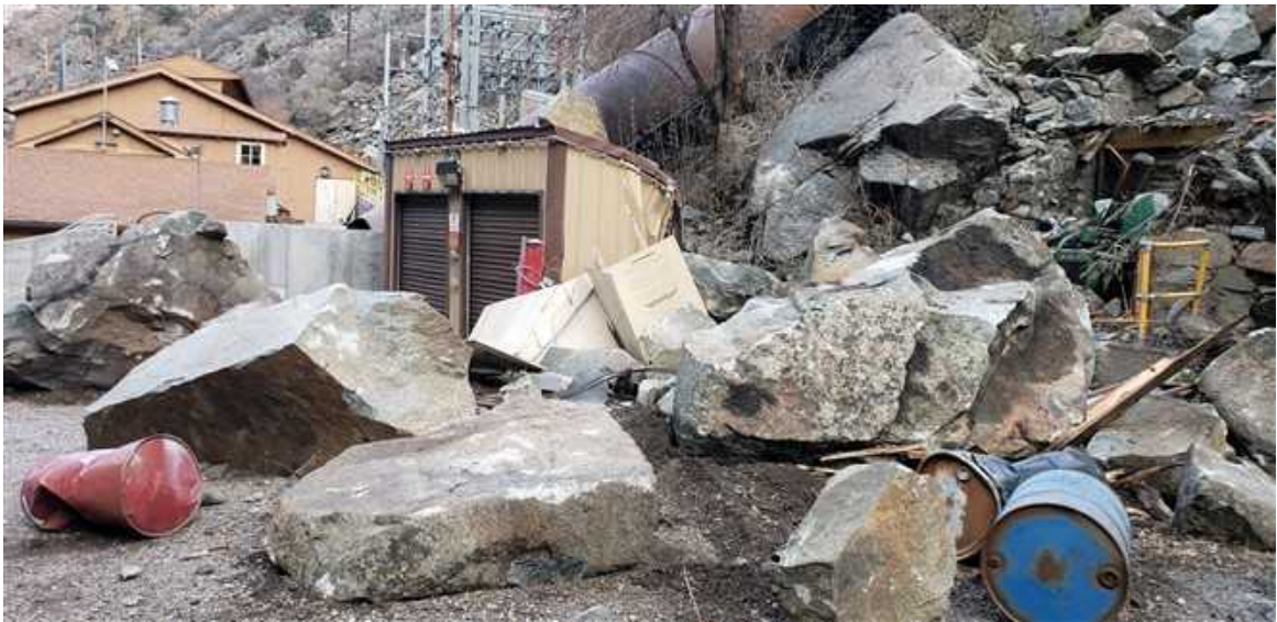
TURBINE HALL DAMAGE FROM PENSTOCK RUPTURE
