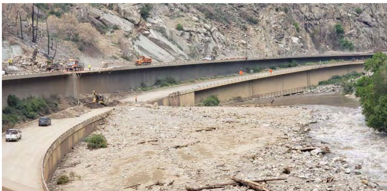
Colorado Department of Transportation crews clear debris and assess damage near Mile Marker 123.5 along Interstate 70 in Glenwood Canyon. Eastbound lanes in the section were destroyed by July 29 mudslides. Photo Credit: Pam Boyd and Post Independent (Boyd, 2021).
