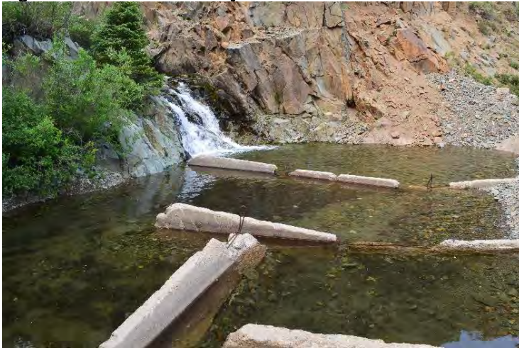
Figure 3-5 Shotcrete spillway and embankment
