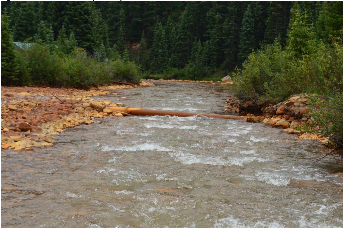
Figure 3-22 Mineral Creek Exposed Pipe
