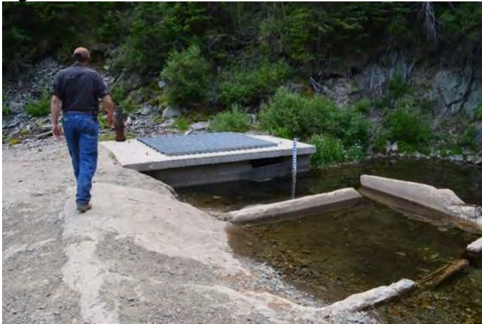
Figure 3-8 Boulder Creek water fall and stilling basin with Baffles
