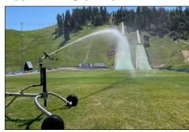
Annual water savings are estimated to be 20% or approximately 11.83 acre-feet in the first full year. This system will allow for automatic daily water adjustments based on real-time weather and soil conditions and will automatically detect water line breaks and shut down water supply immediately.
