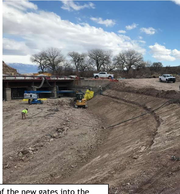
Right: Installation of one of the new gates into the Gunnison River Diversion Structure Left: Grading of the Power Canal
