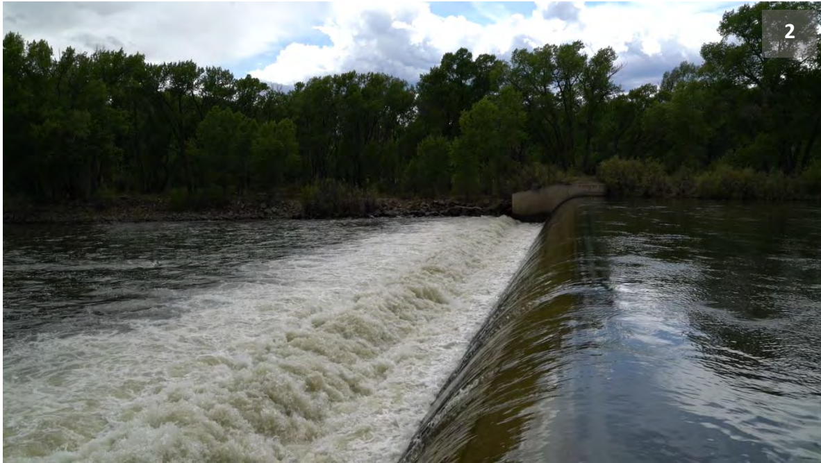
Photo 2. Hydraulic jump created by Rio Grande Canal low head dam structure.
