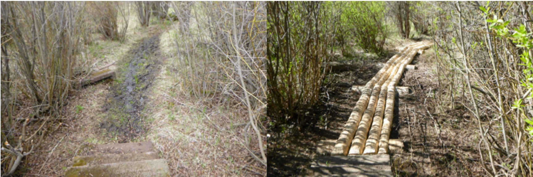
Figure 4. Pre/post photos (above and below) showing puncheon structure constructed by RMFI crews in 2021 to mitigate erosion and create a more durable trail surface.
