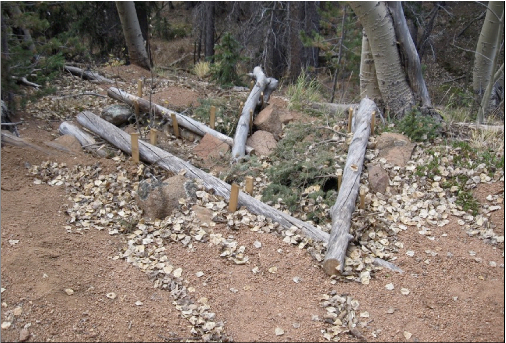
Figure 5. Example of a brush filter constructed between the trail and Bear Creek to help capture sediment.
