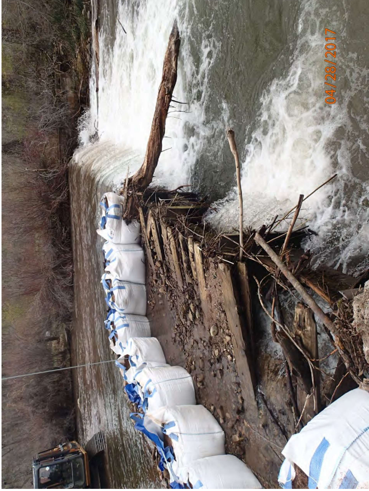
Photo 3: Florida Canal Diversion Structure - Emergency Repair 2
