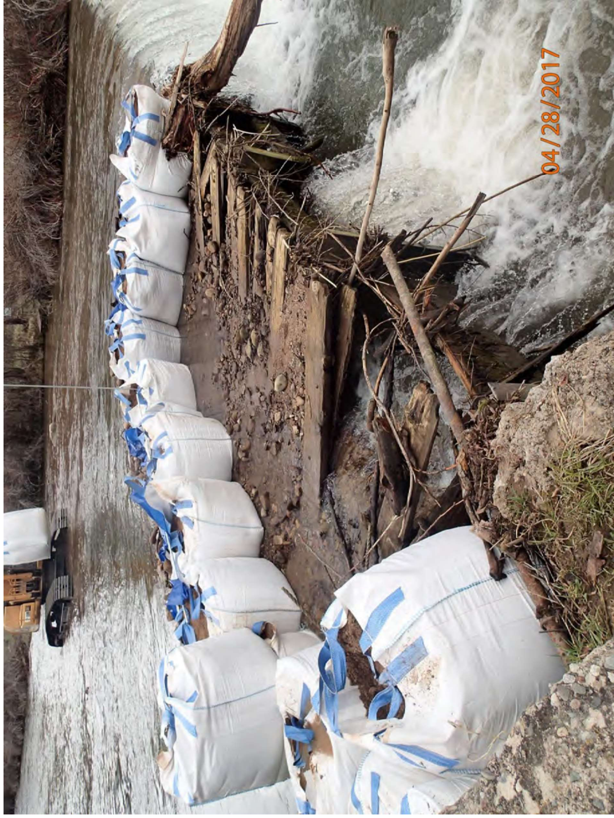
Photo 2: Florida Canal Diversion Structure - Emergency Repair
