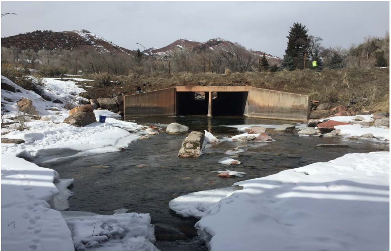
Canyon Creek Culvert under Interstate 70. Looking north, April 2019.
