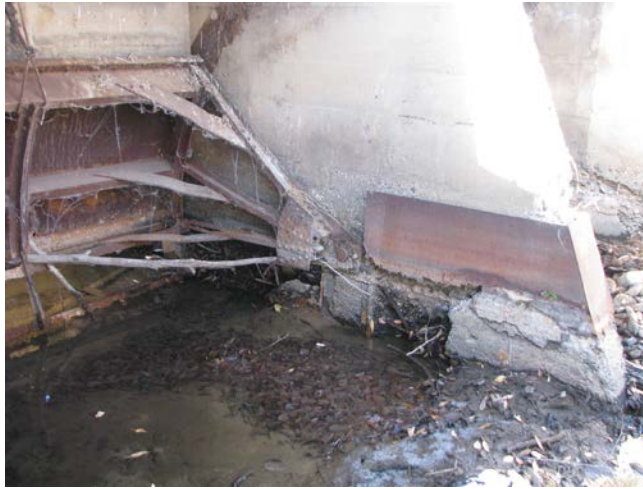
Main Canal Head gate showing deterioration from corrosion
