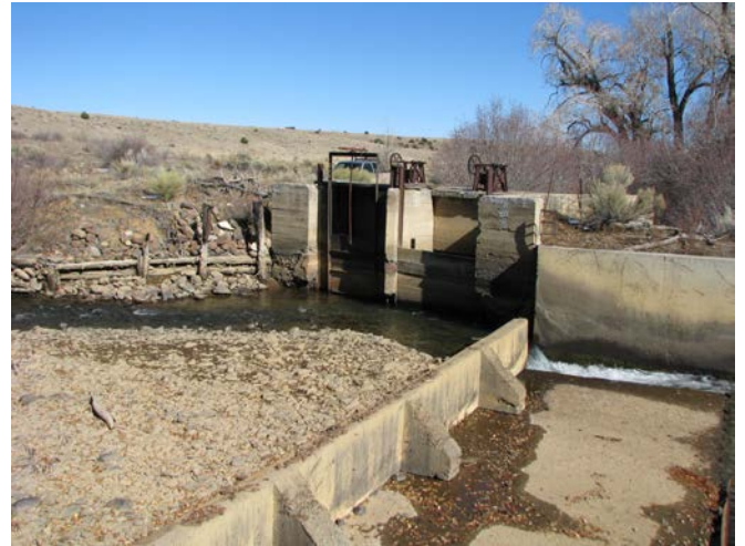
Main Canal Head gate showing deterioration from corrosion
