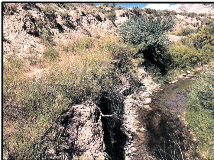
Parachute Creek undercutting nearing Diamond Ditch embankment. Ditch to be re-aligned away from creek.
