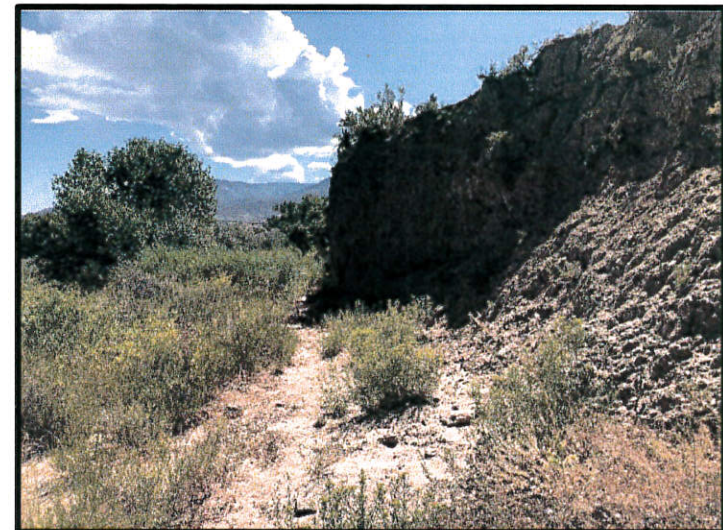
Steep bank overhanging (shown on right) Diamond Ditch alignment (located in willows shown on the left). Ditch maintenance has been deemed hazardous due to threatening sheer slope.
