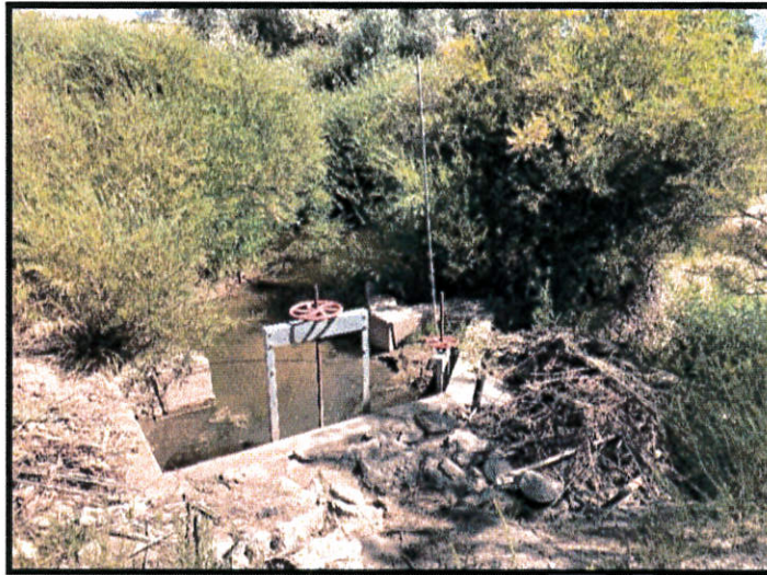
Diamond Ditch Headgate. Replaced in 2016
