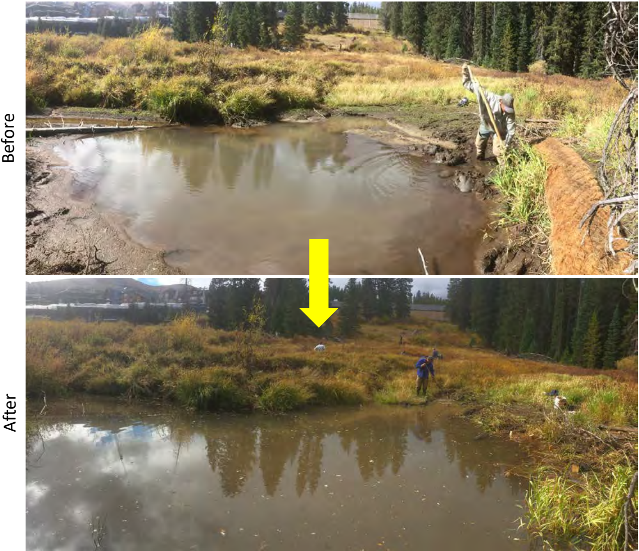
↑Repairing breached beaver dams with coir logs and sod.
