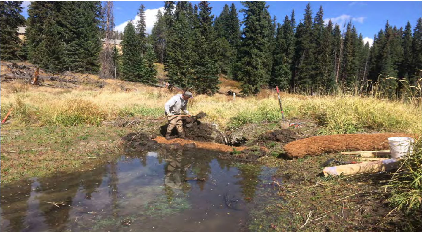
↑ Repairing breached beaver dams with coir logs and sod. ↓ Before and after.
