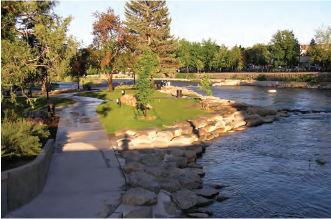
Bank Stabilization & Improved River Bank Access
