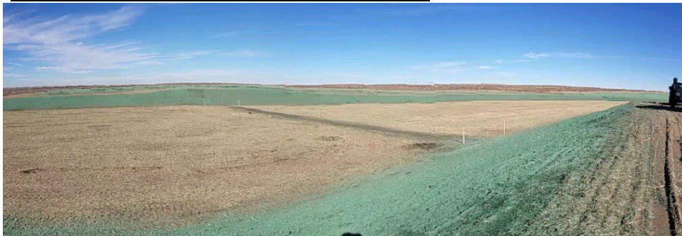
ACB mat installation at Station 17+00 completed. Mat joints still require concrete fill.
