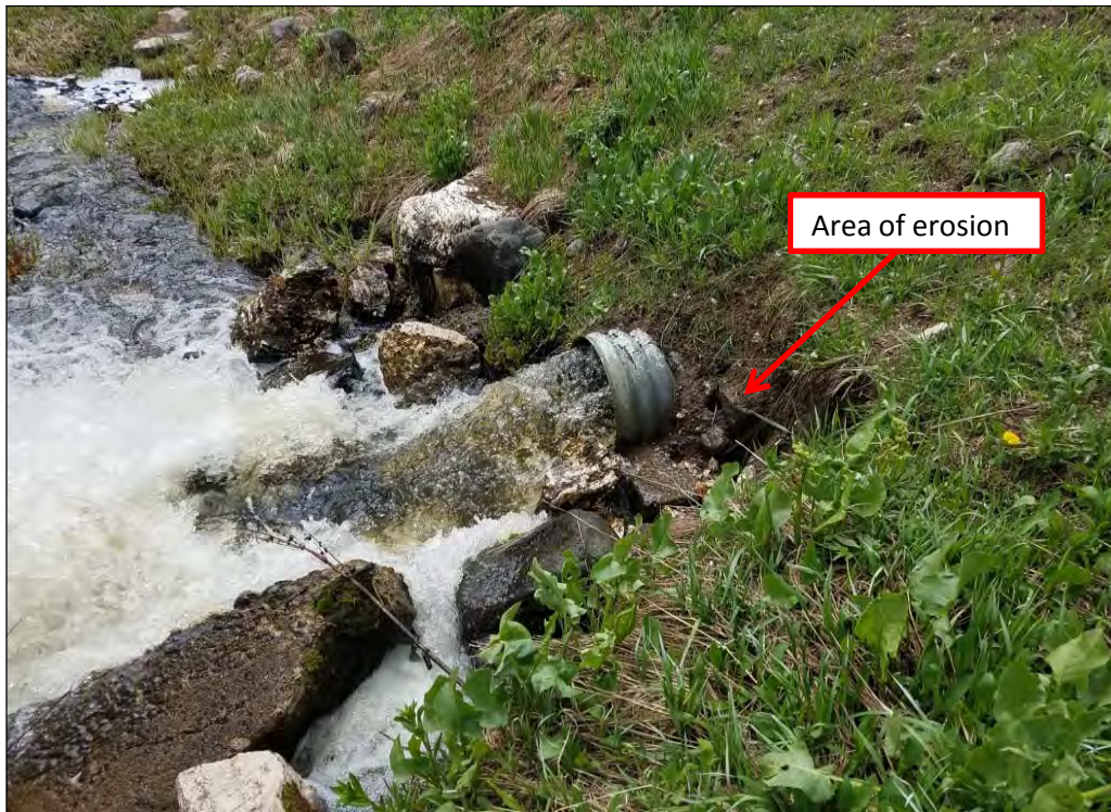
Outlet pipe flowing full at time of inspection. Note area of erosion on left side of pipe.
