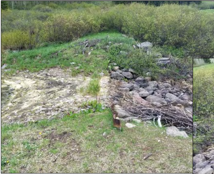
Spillway has some wood debris and brush encroaching on the channel.
