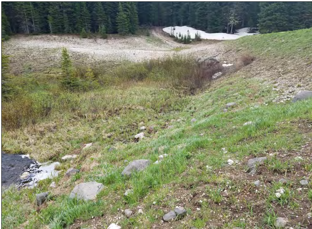
Downstream slope is steepened on right side of dam.
