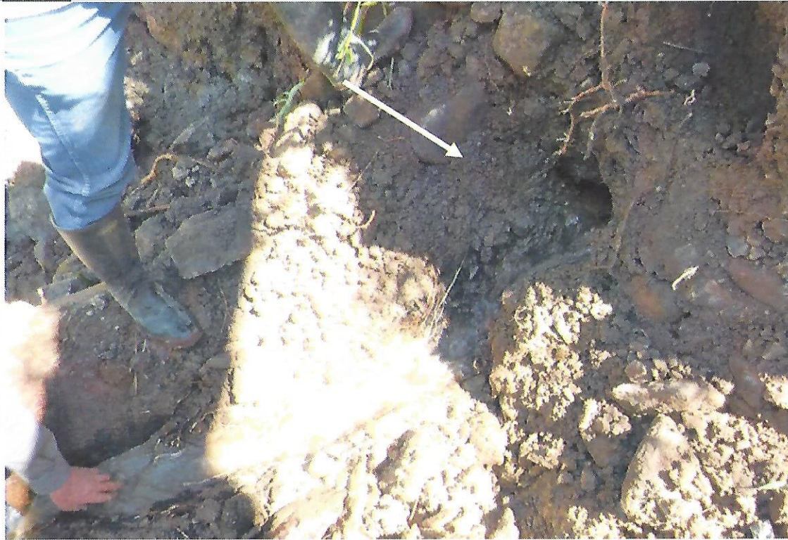
Photo supports well-defined concentrated exit point indicating possible erosion pipe formation (ADVERSE FACTOR).
