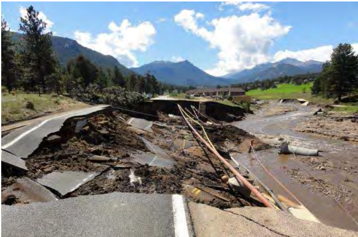
Flood damage to roads exposed the utility lines in 2013 (photo by Water Quality Control Division staff).
