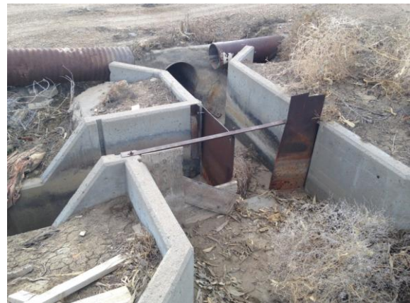
Divider box on the lateral serving the Hanagan Recharge Pond
