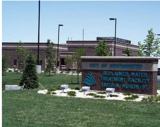
Figure 4: City of Westminster Reclaimed Water Treatment Facility
