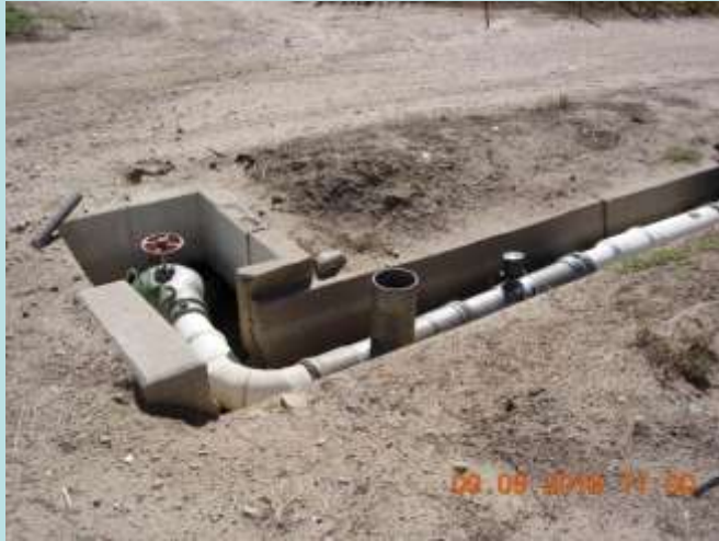
Field inflow meter and RO ramp flume
