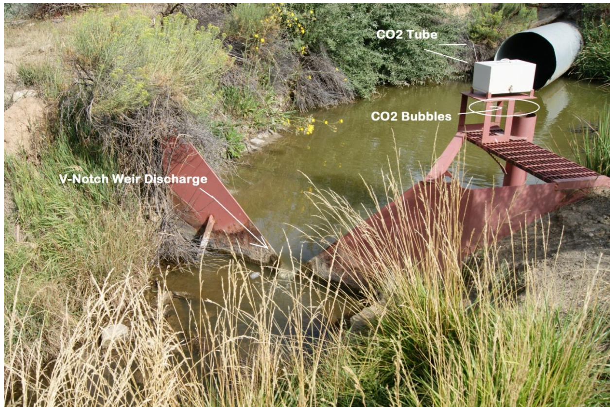
Photo 3 – Pond 007 discharge pool
