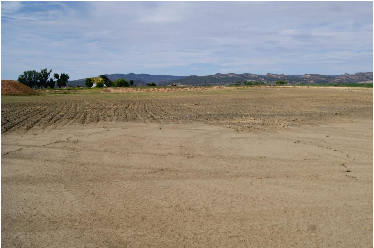
Photo 10 – Surface roughening on Morgan spoil, looking SW
