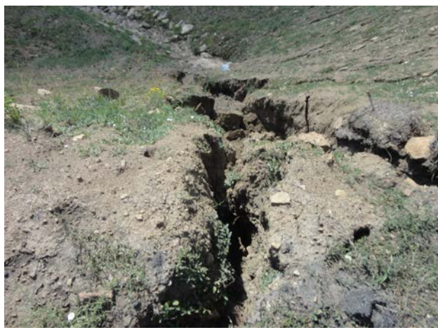
Photo 8: Erosion above pond 8
