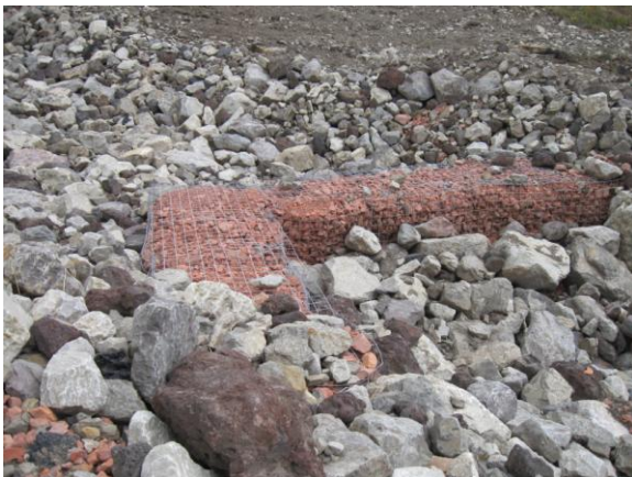
Gabion installed
