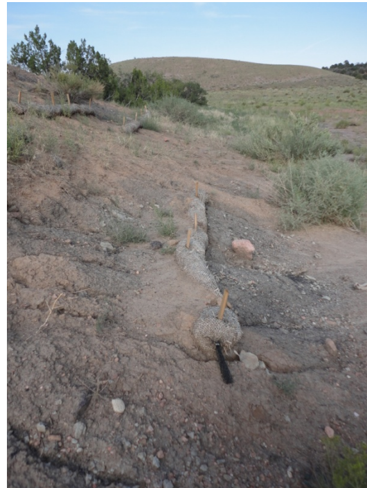
Photo 8: wattles stabilizing slope.
