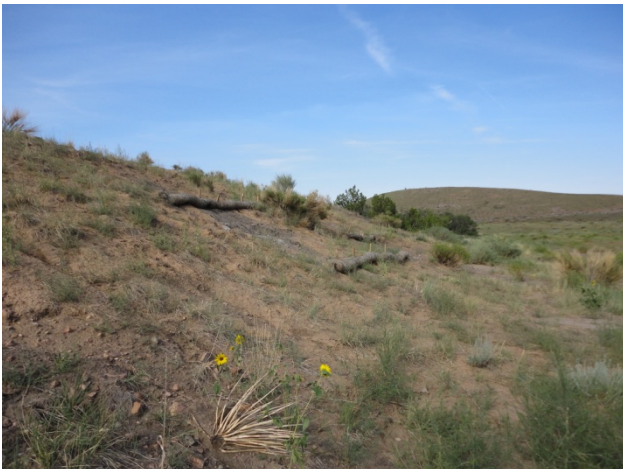
Photo 7: effective wattle placement on slope north of permanent parking area.
