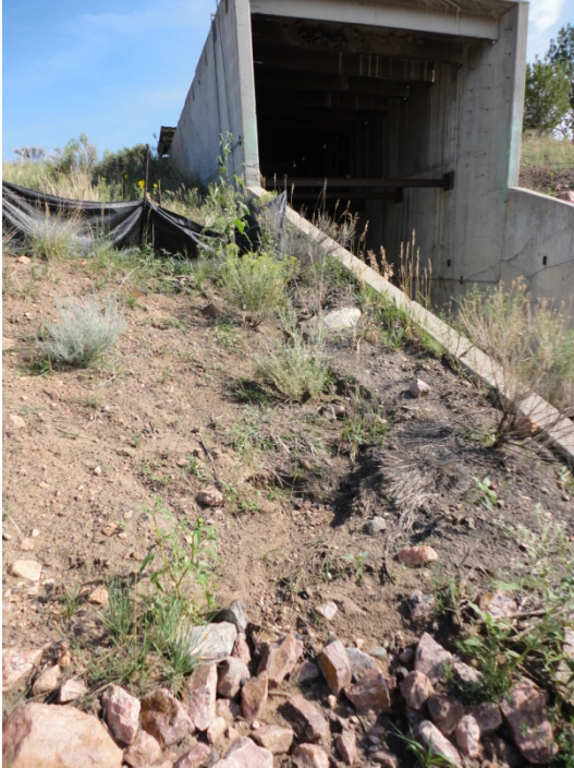
Photo 5: rill repairs adjacent to truck tunnel holding well but poor seedling emergence
