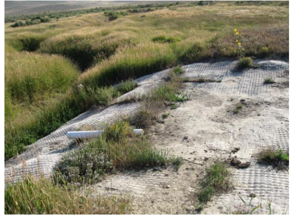
Rail loop pond spillway. Earth berm needs repair.
