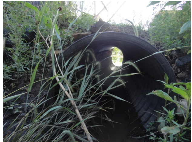
Photo 60: C17A partially backed up
