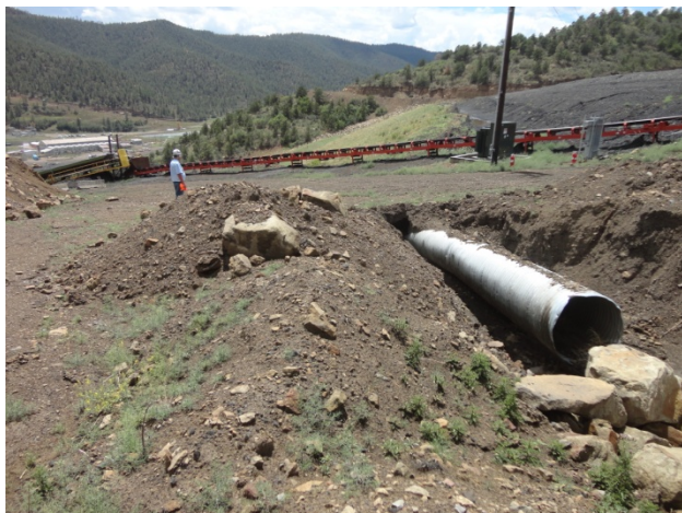
Photo 37: Unidentified and damaged culvert on east side of RDA
