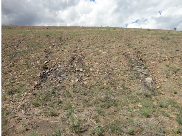
Photo 43: Erosion on DWDA 1 to be repaired
