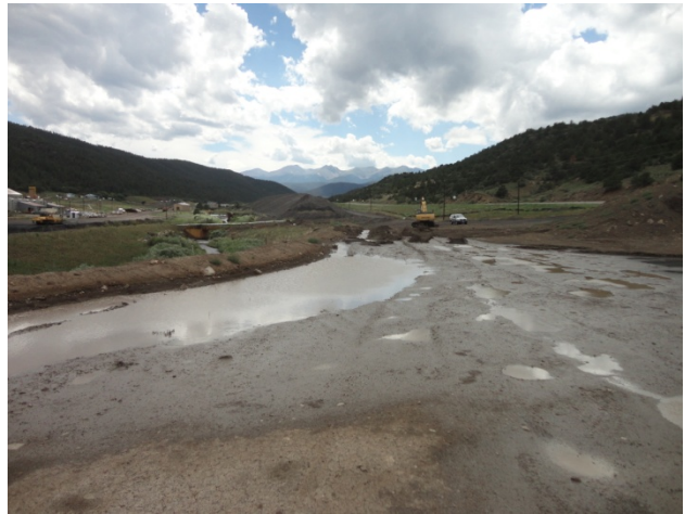
Photo 46: SAE showing berm and high spot to be graded out
