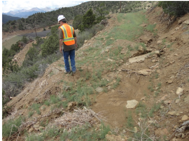
Photo 34: Erosion below cell phone pad (1)
