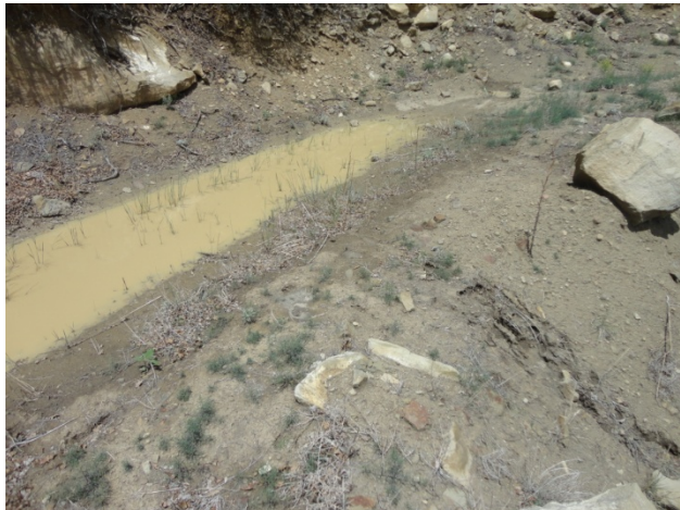
Photo 33: Low spot and breach in RDA diversion ditch, to be surveyed
