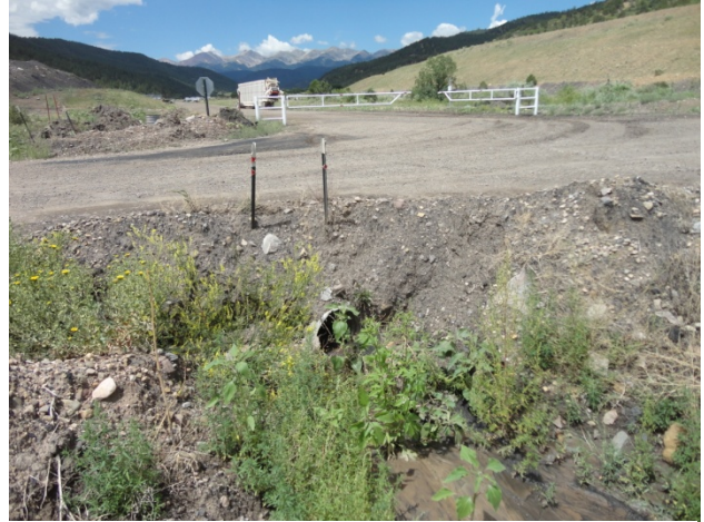
Photo 26: C9 to be cleared at outlet
