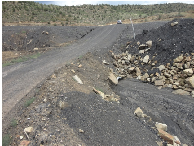
Photo 29: Culvert under road on west side of RDA to be cleaned
