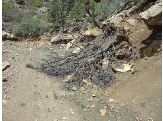
Photo 32: RDA diversion ditch to be cleared
