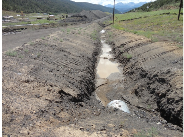
Photo 44: New culvert (C14?) to be cleaned
