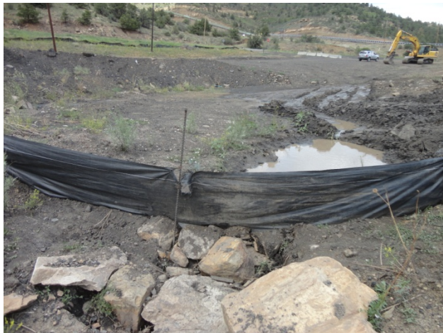
Photo 47: Silt fence at west end of SAE
