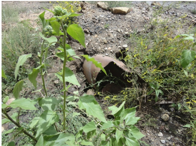
Photo 27: C8 inlet damaged
