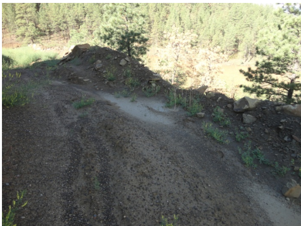
Photo 5: Low spot in water tank SAE berm
