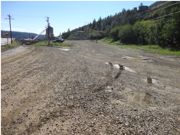
Photo 65: New drainage scheme needed around East Portal fan
