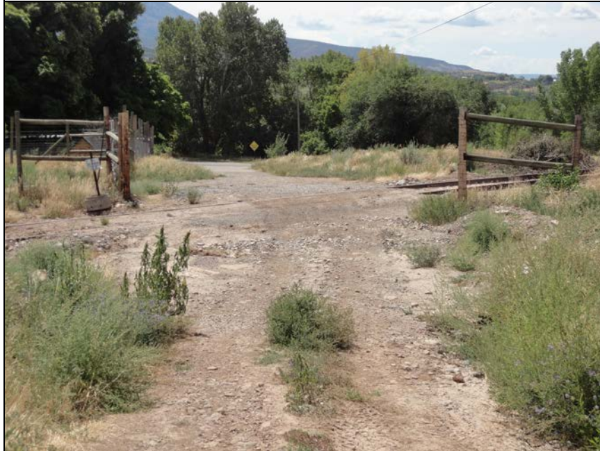
Photo 15 Loadout gravel storage area SAE – berm should be parallel to tracks, on near side
