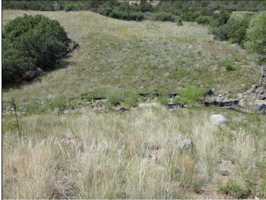
Photo 14 Silt fence on Stevens Gulch at ROM area
