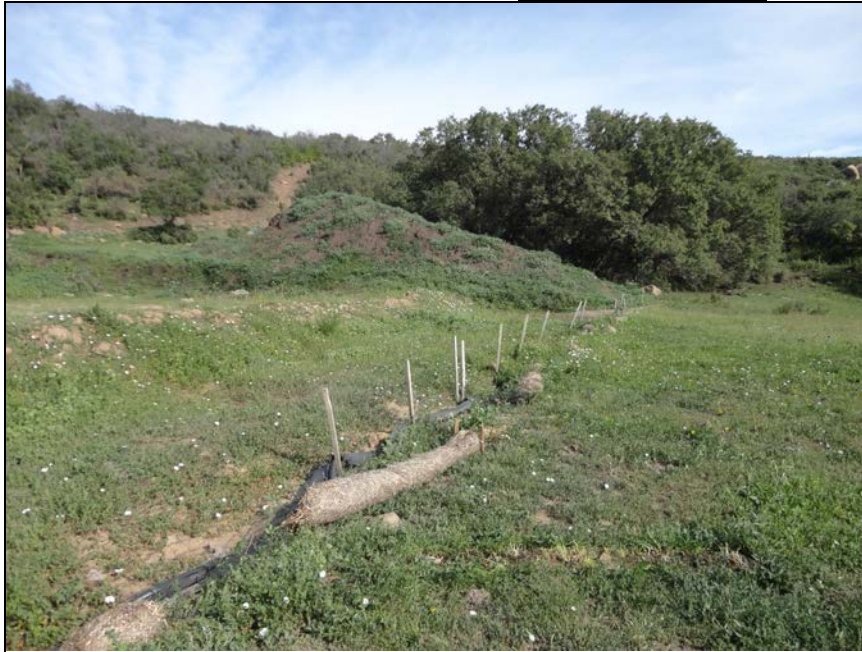
Photo 1 GVB – B12C drill pad, straw wattles have been damaged by cattle
