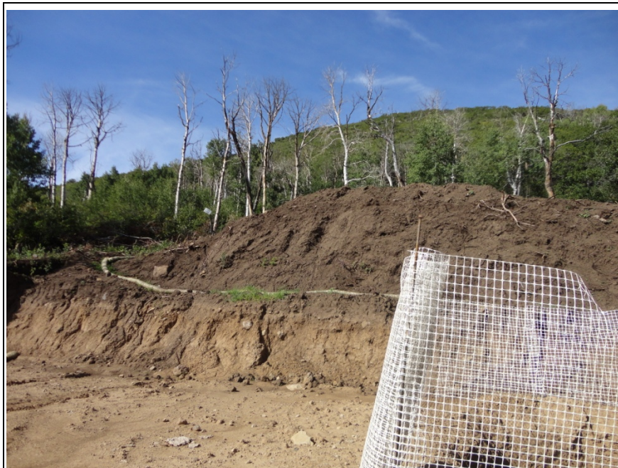
Photo 3 Topsoil stockpile and excavated bench at GVB – B14C
