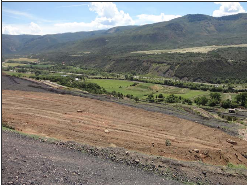
Photo 10 Cover material on Gob Pile #4
