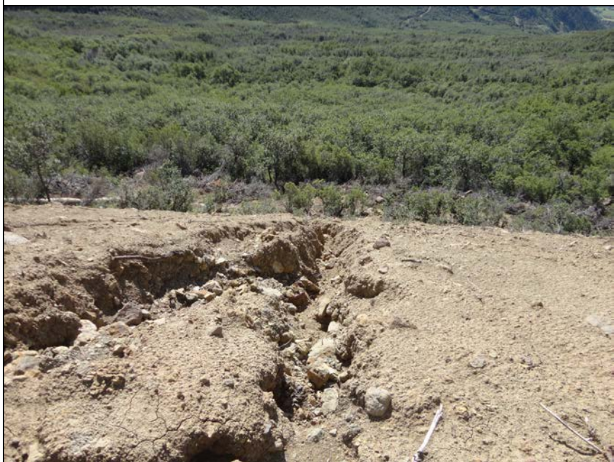
Photo 4 Outslope of GVB – B14A, where berm was low
