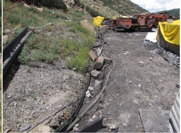
Photo 2 – Ditch D3 Needs to be Cleaned
