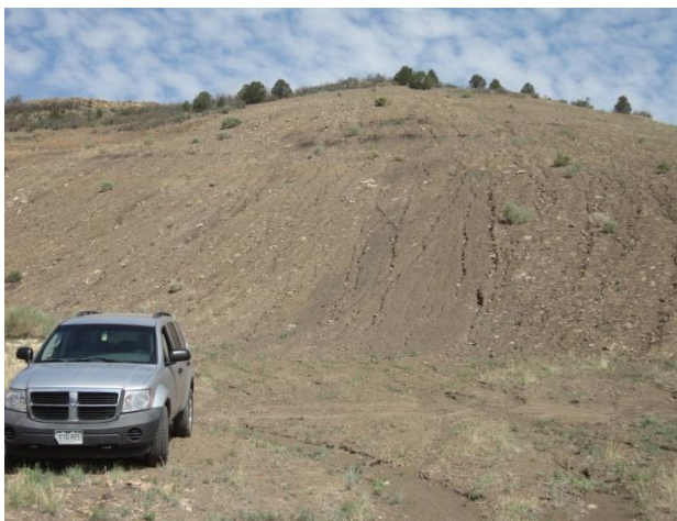
Photo 34: Steep slope above pond 6, showing erosion (1)
