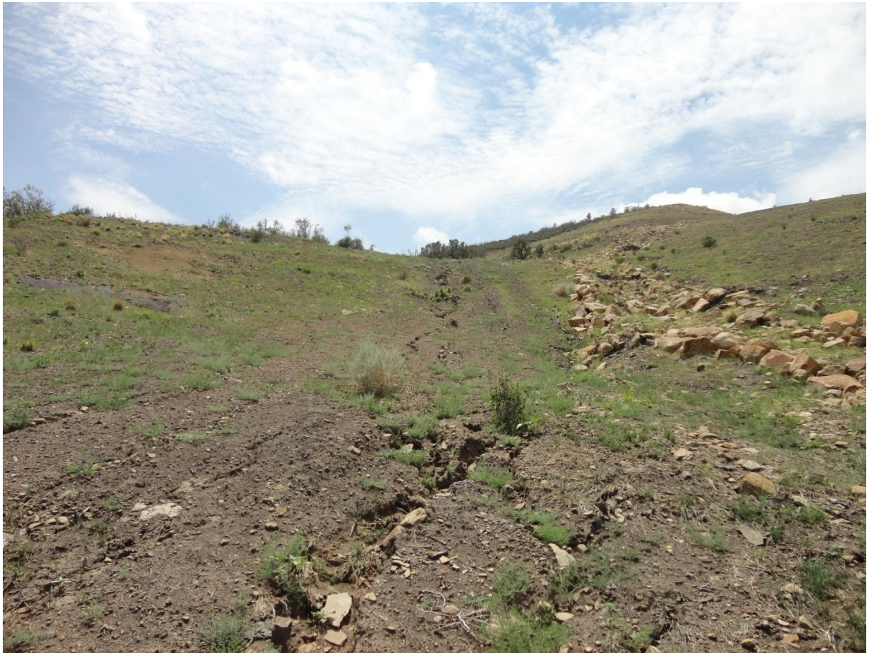
Photo 45: Erosion outside of fill 8 (2)
