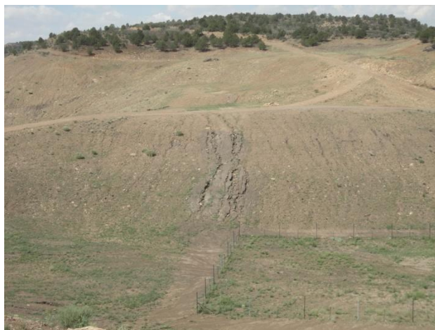
Photo 37: Steep slope above shrub plot, showing erosion
