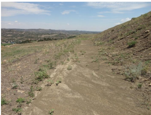
Photo 49: Sediment in contour ditch north east of "nob"
