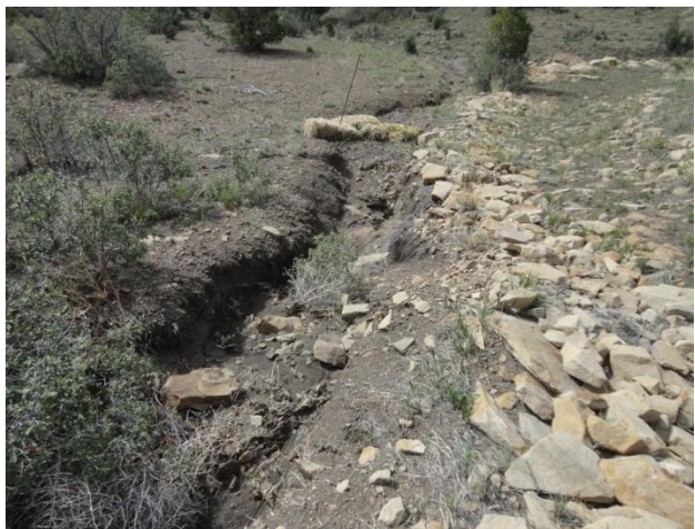
Photo 29: Erosion next to pond 6 emergency spillway (4)
