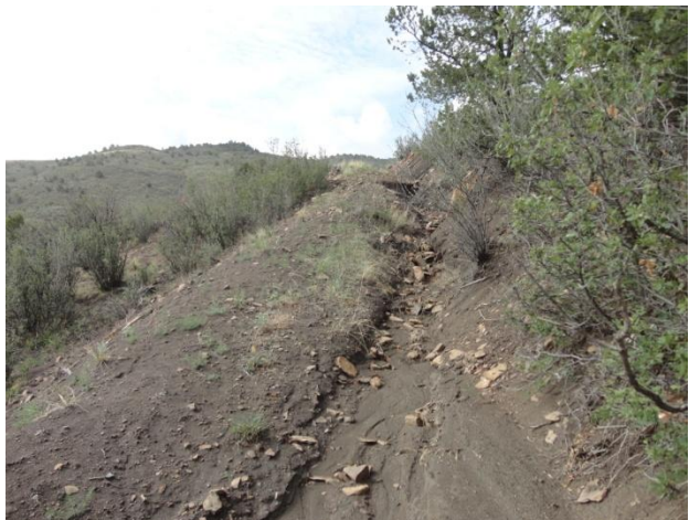
Photo 19: Contour ditch west of fill 7 to be cleaned (1)
