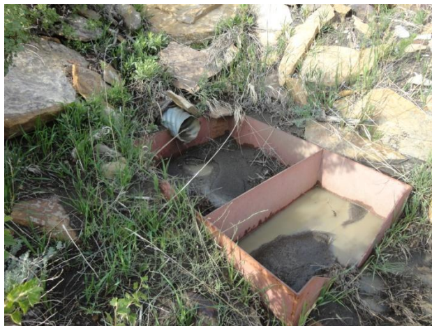
Photo 3: Pond 9B weir box
