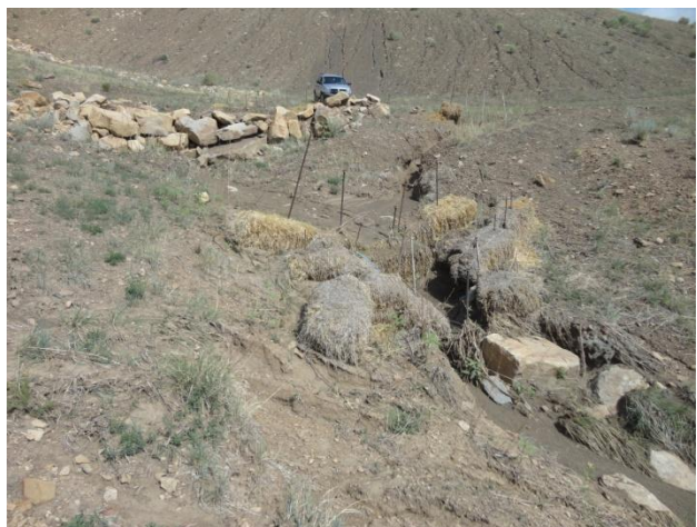
Photo 33: Accumulated sediment above pond 6 (4)
