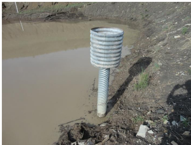
Photo 4: Pond 9B primary spillway riser
