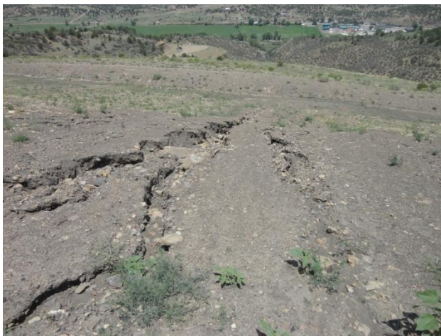
Photo 51: Erosion north east of "nob" (2)
