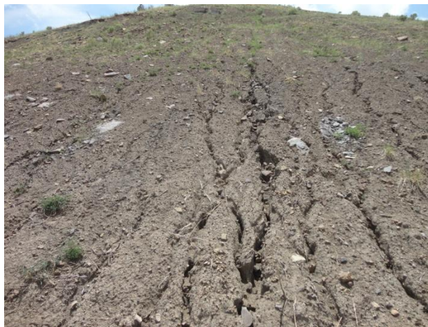
Photo 50: Erosion north east of "nob" (1)
