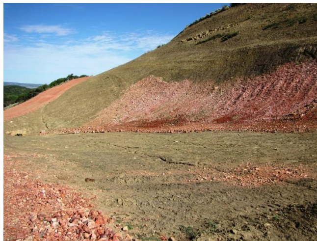
Slide damaged area above Pond 016
