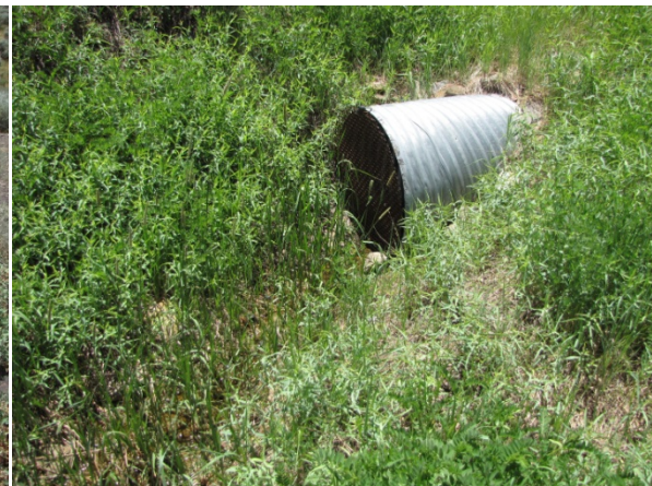
Photo 4 – Fan Shaft Access Culvert is Seeping Water
