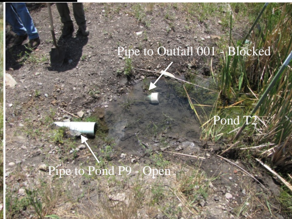
Photo 2 – Diversion Structure at Pond T2 Outlet
