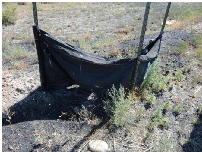
Silt fence at west end of loadout
