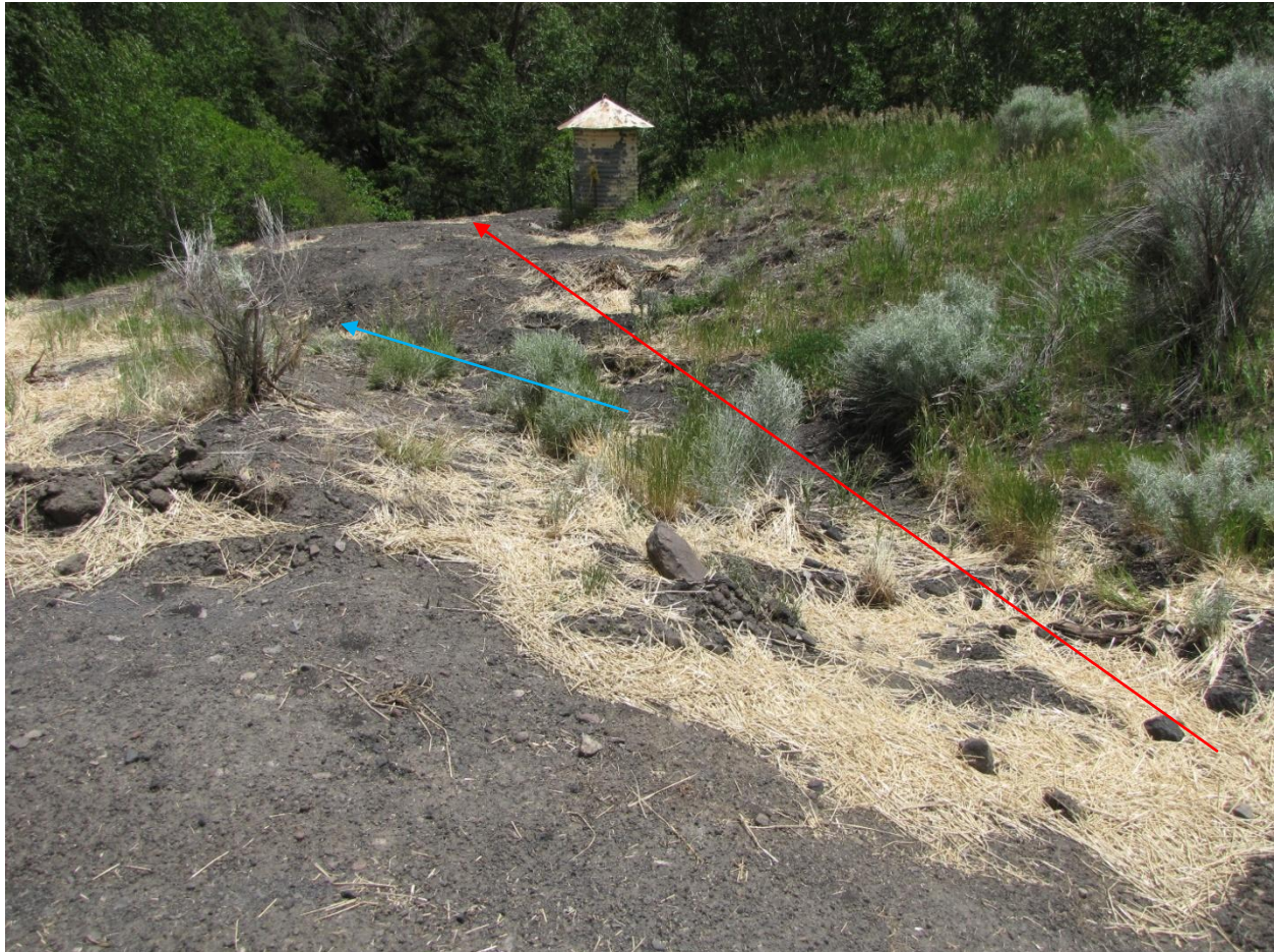
Photo 4 – The red line shows the location of the permitted emergency spillway ditch, which has been filled in. The blue line shows the direction of the current ditch directing water to the Refuse Pile Pond Ditch.
