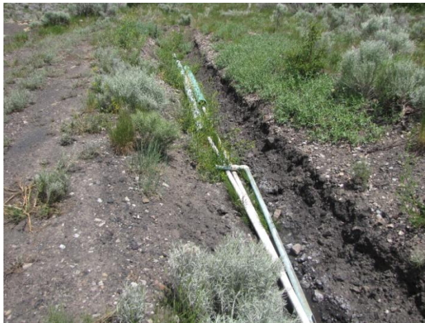
Photo 5 – Pipes in Ditch Need to be Removed
