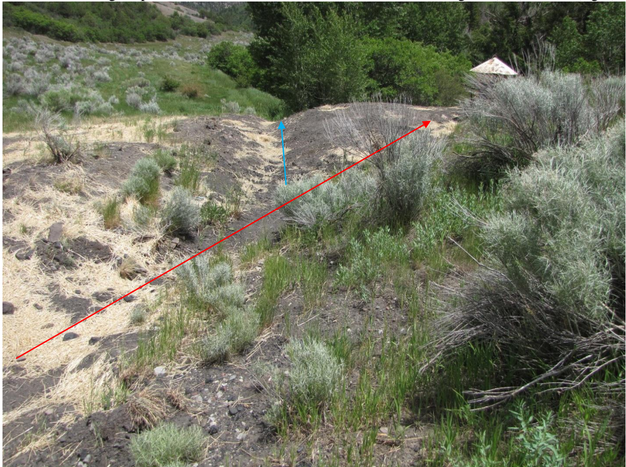
Photo 3 – The red line shows the location where the permitted emergency spillway ditch is supposed to be. The blue line shows the current ditch directing water to the Refuse Pile Pond Ditch.
