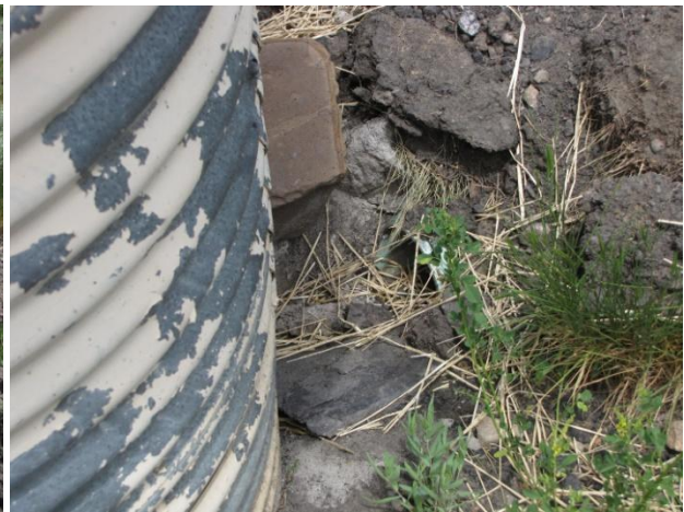
Photo 6 – Outlet Pipe Needs to be Cleaned
