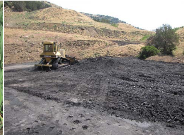
Photo 4 - Coal Waste Being Spread Into a Lift
