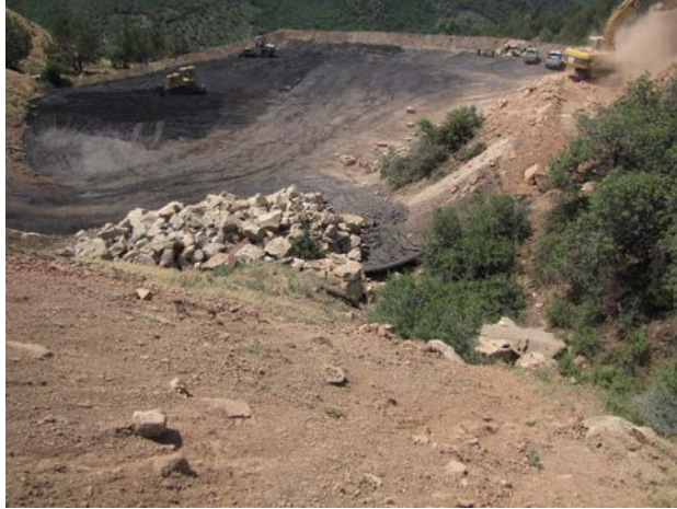
Photo 7 – Underdrain Construction
