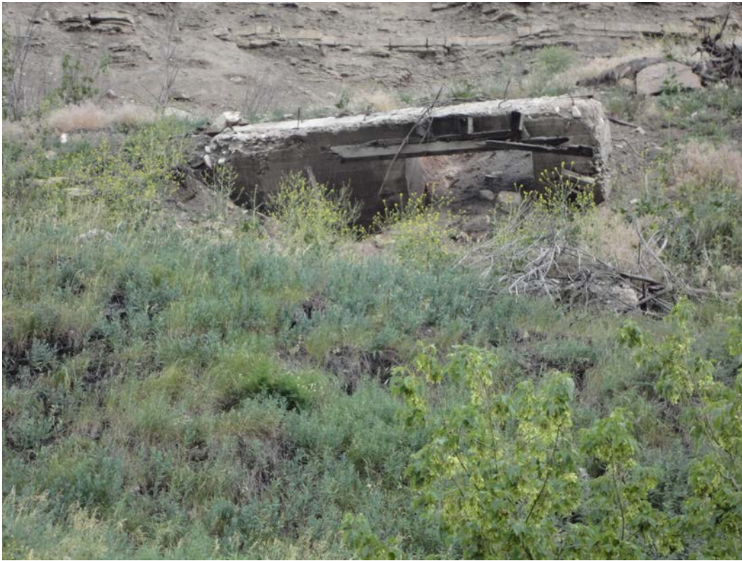
Concrete abutment protruding from backfill
