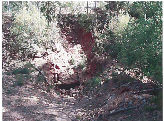
Figure 14: Chief Tunnel collapsed opening.
