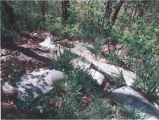
Figure 19: Sand bags utilized for sediment detention structures along access roads are deteriorating and sliding down slope.
