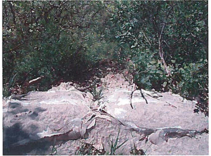
Figure 20: Sand bags utilized for sediment detention structures along access roads are deteriorating and sliding down slope.
