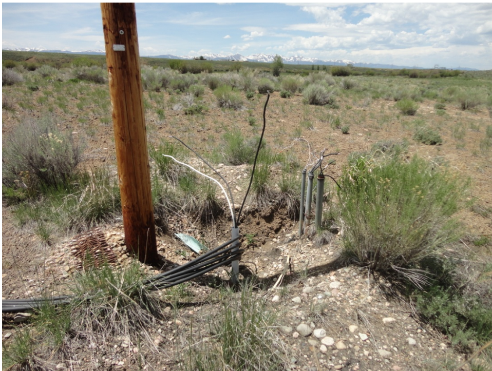
Photo 4: Bare cables at the loadout
