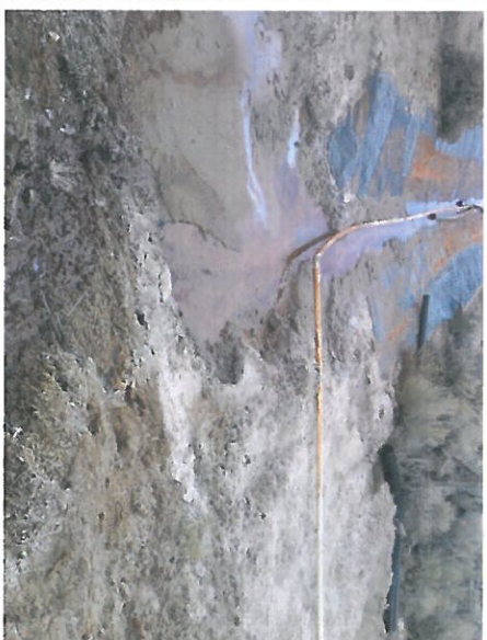
Photo 8 – Seepage at toe of the main dam. Majority of seepage comes through collection drain, but some seepage appears to be uncontrolled (see Photo 9).
