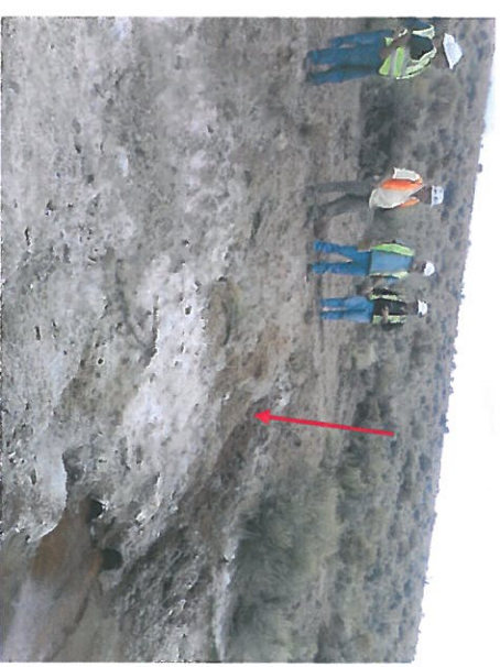
Photo 9 – Seepage drain outfall at the downstream toe (3x12" HDPE pipes). There is reportedly a large seepage collection pipe under the dam. NOTE: Uncontrolled seepage exiting higher on the slope above the drain outfalls (red arrow).
