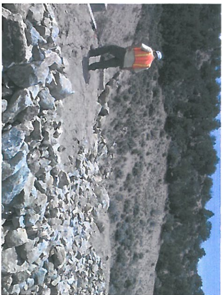
Photo 7 – Recent erosion repairs performed around the south diversion drop structure outfall.
