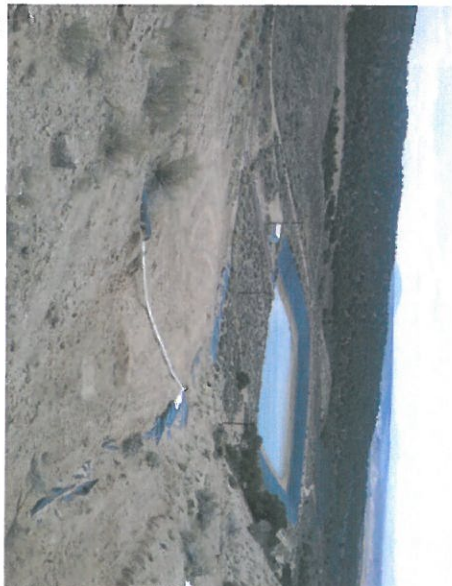
Photo 5 – Foreground shows right groin where liner and erosion damage was recently repaired. Background: seepage collection pond at the downstream toe of the main dam.
