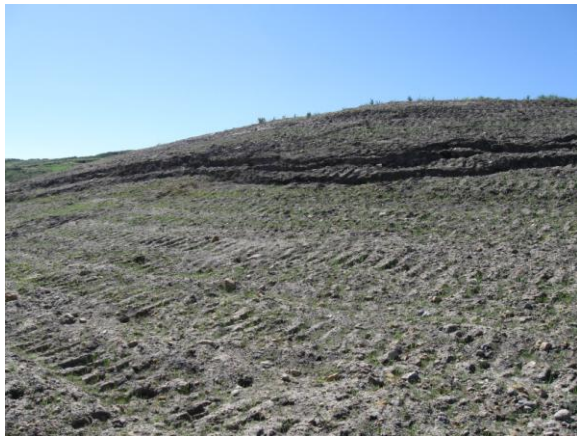
Parcel E-AB-08; Slump Area above D Pit. Recent settling cracks.
