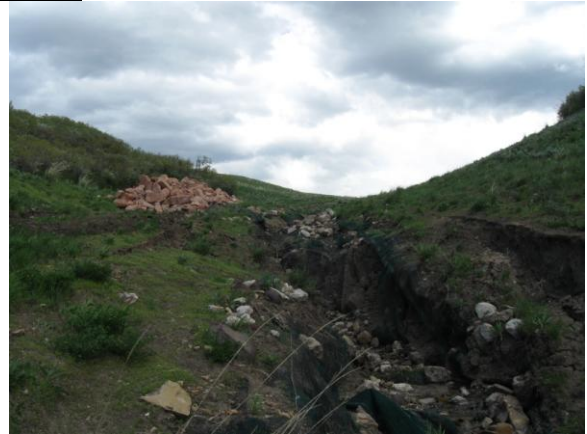
YPM-6-1, riprap stored adjacent to the channel.
