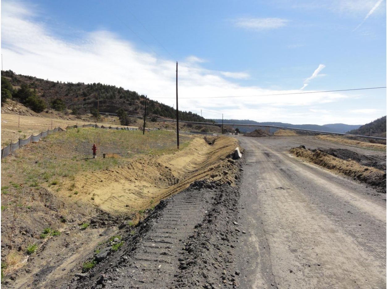
Hydroseeding at ditch D-19
