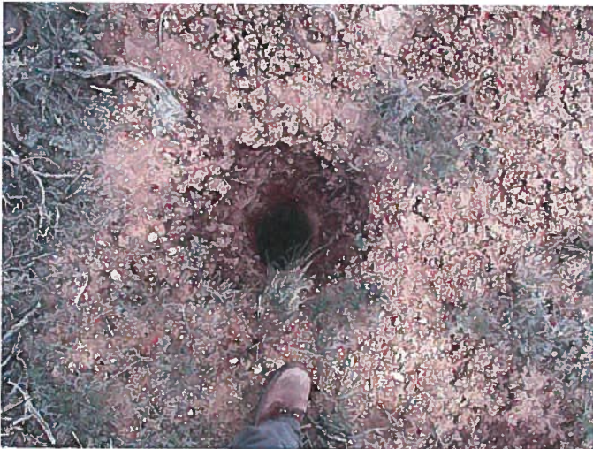
Figure 11: Unreclaimed auger hole located just beyond the stormwater berm on the northeast side of the disturbed area.
